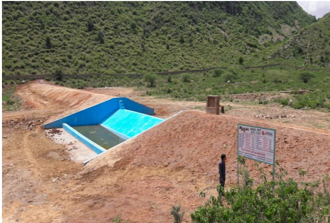
Check dam constructed under Krishi Jyoti Project
