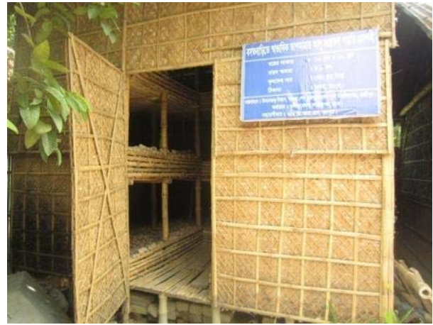
Potato storage structure for village conditions developed and promoted by RDRS in Rangpur district of Bangladesh
